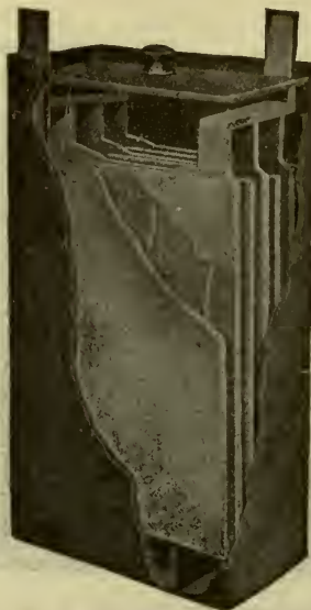
FIG. 427.—One Cell of the "Gould" Storage Battery for Electric Vehicle Use. According to the data given by the manufacturers, this cell, containing four negatives and three positive plates, has a normal charging rate of 27 amperes; a distance rate of 22\frac{1}{2} amperes for 4 hours; a capacity of 81 ampere-hours at 3 hours' discharge, and of 90 ampere-hours at 4 hours' discharge. The plates are each 5\frac{7}{8} \times 7\frac{3}{4} inches, and the total dimensions of the cell, enclosed in its rubber jar, are 2\frac{1}{2} \times 6\frac{1}{4} \times 11 inches. Forty such cells are generally used for an average light vehicle battery.
